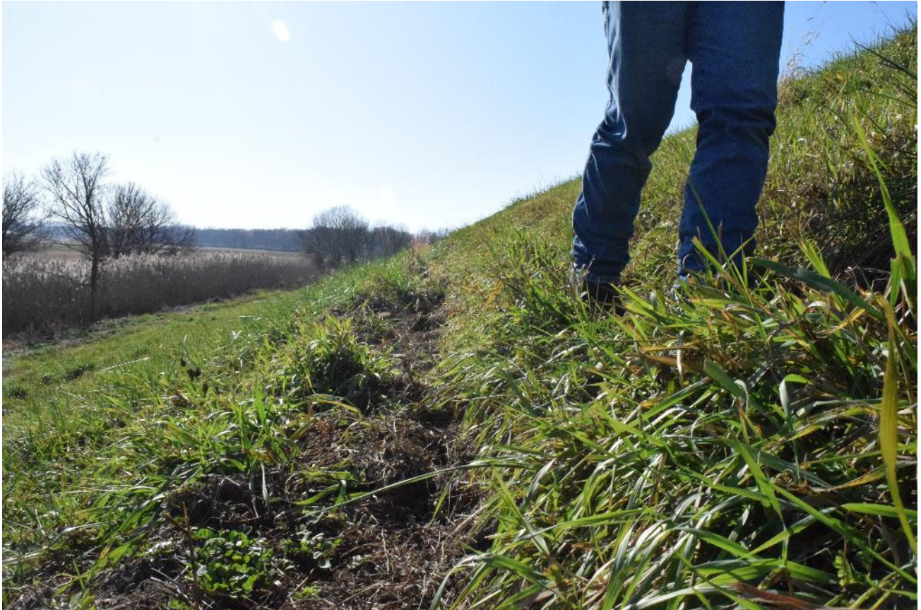
East side downstream slope – repair minor rutting
