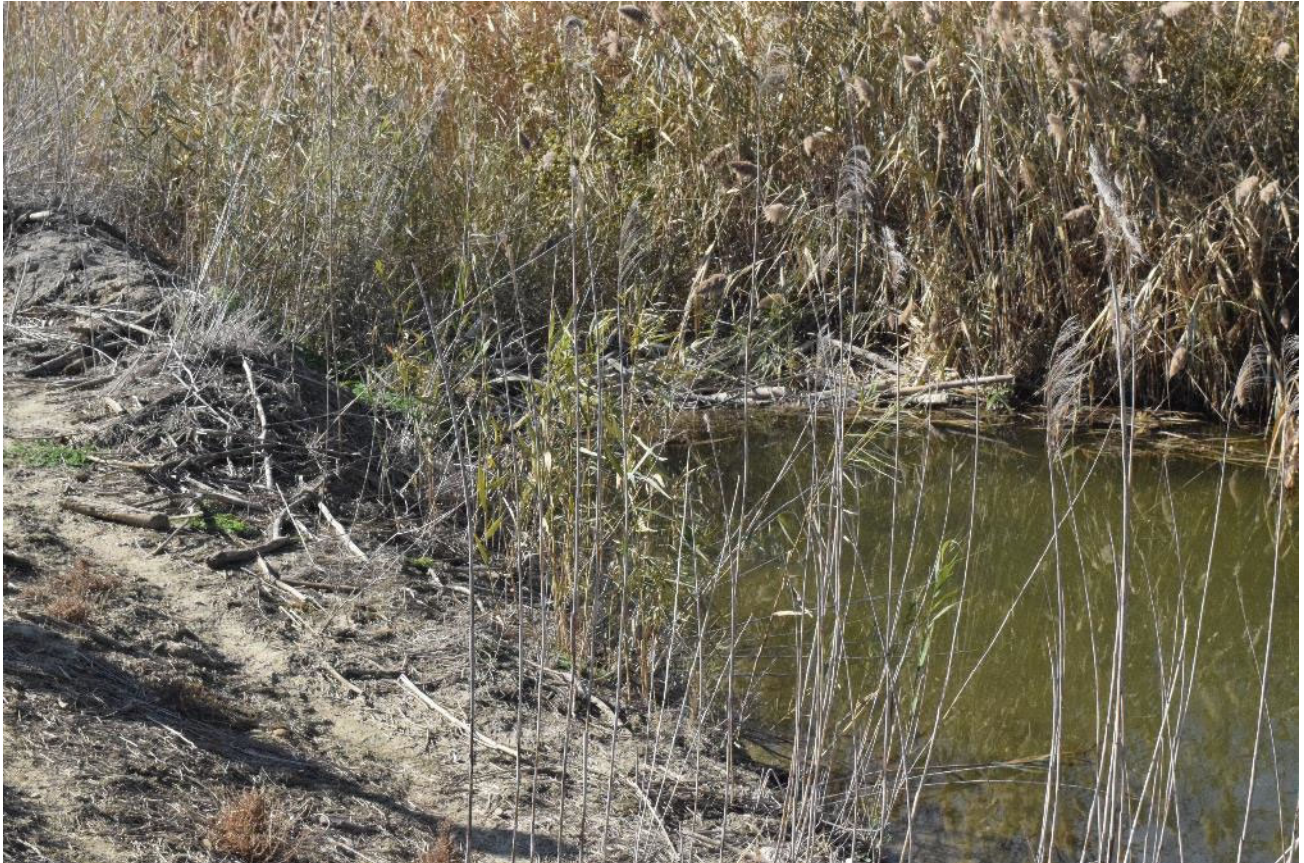
West side ditch – remove dam
