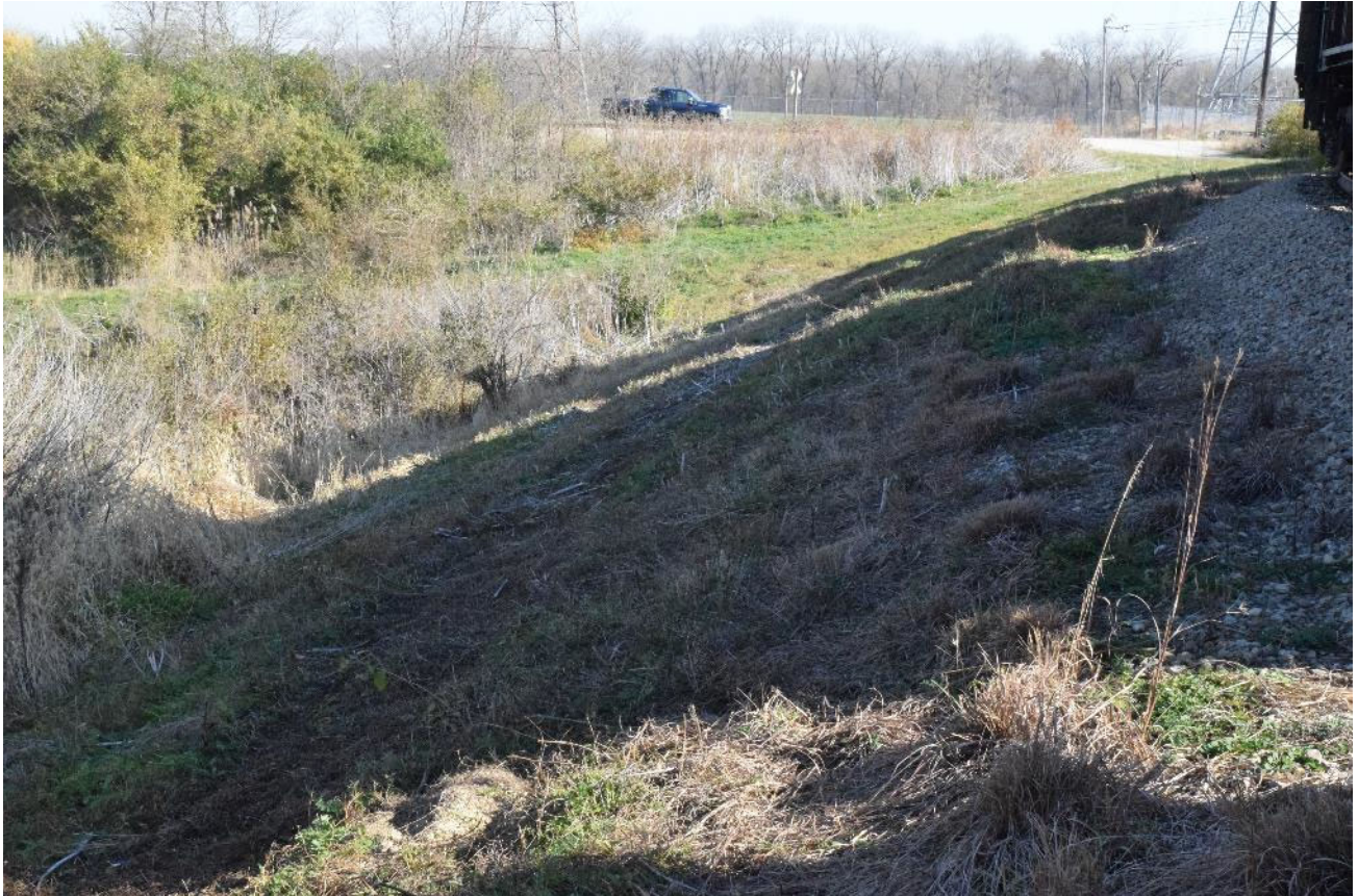
North side downstream slope
