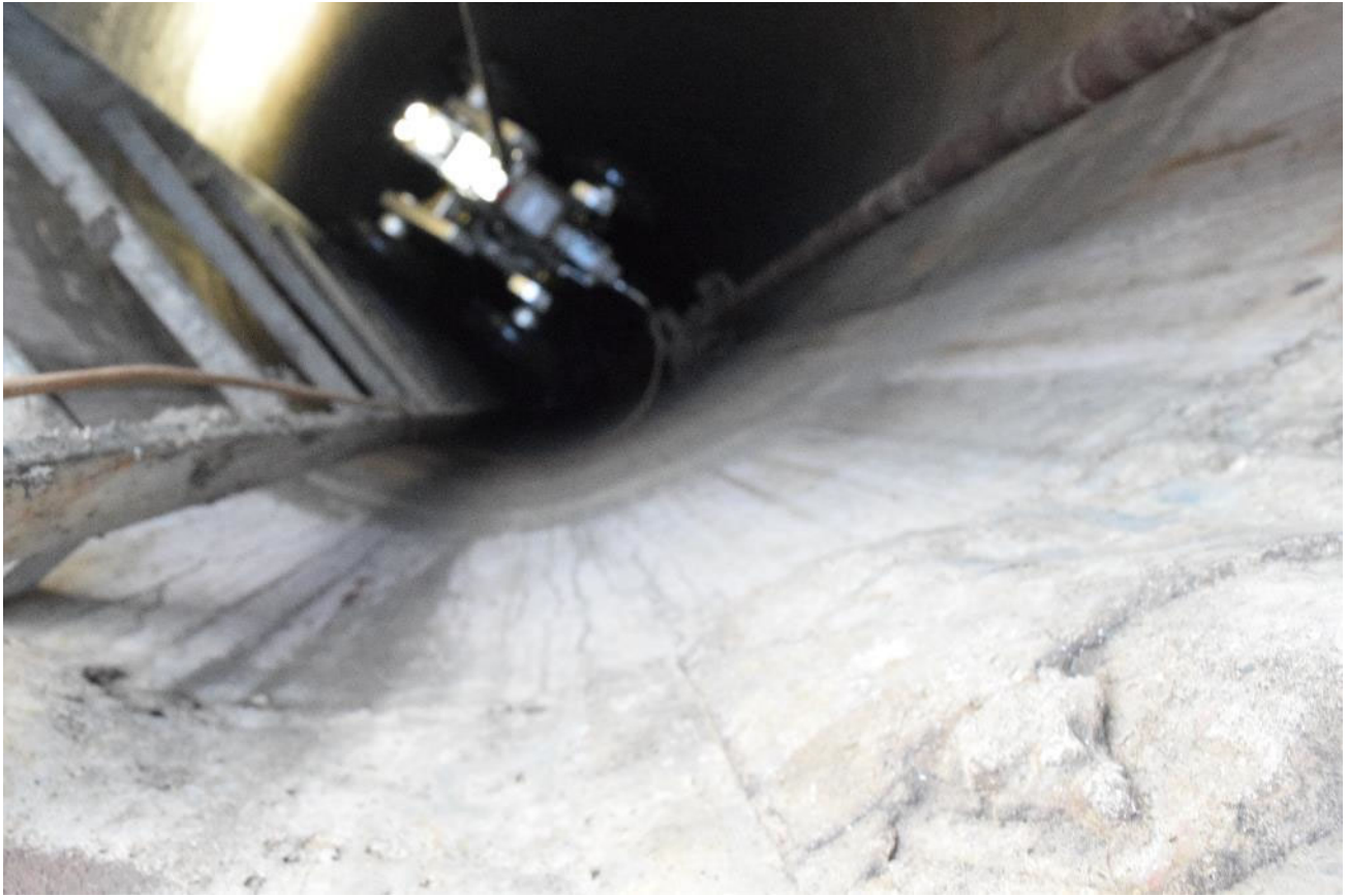
Outlet gate structure at Illinois River
