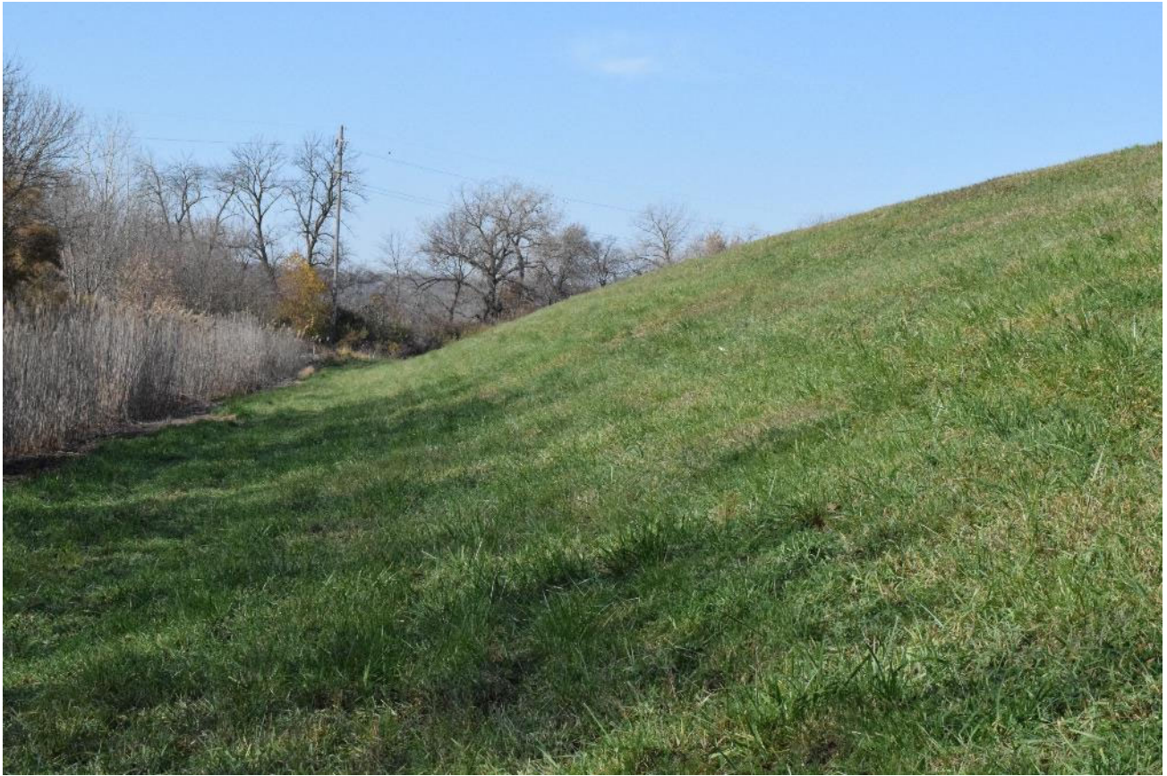
South side downstream slope
