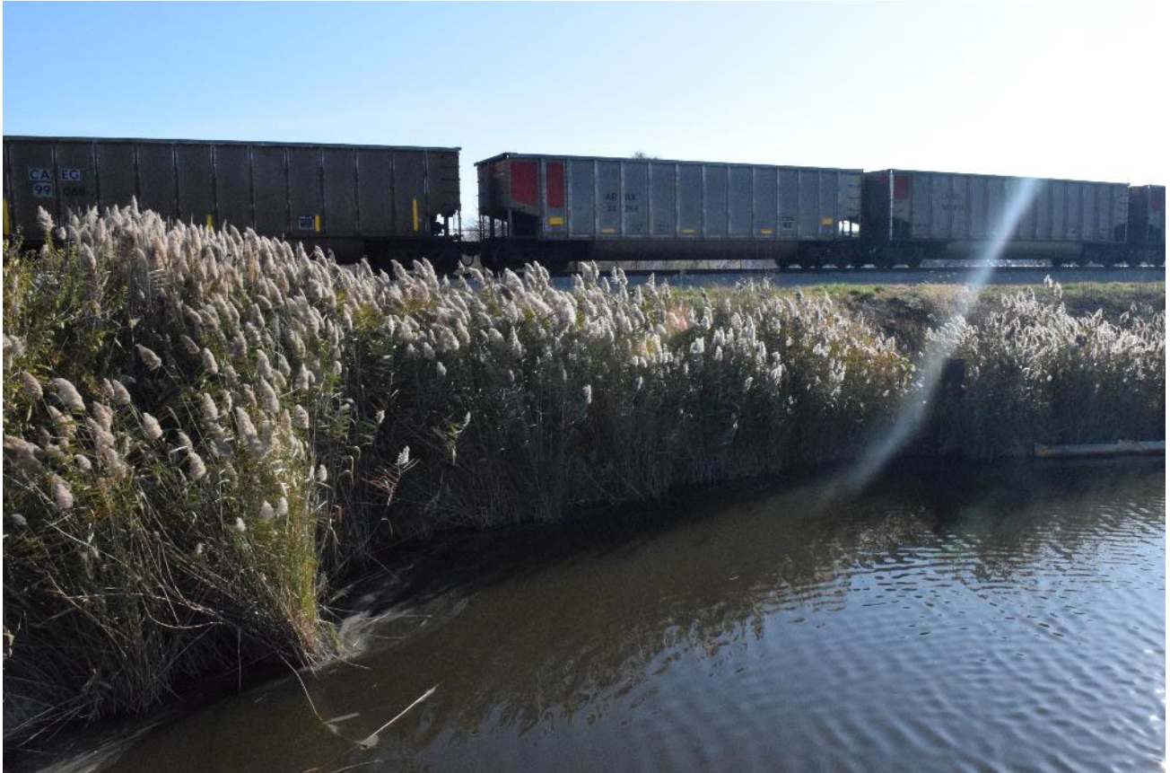
East side upstream slope – spray/remove thick vegetation
