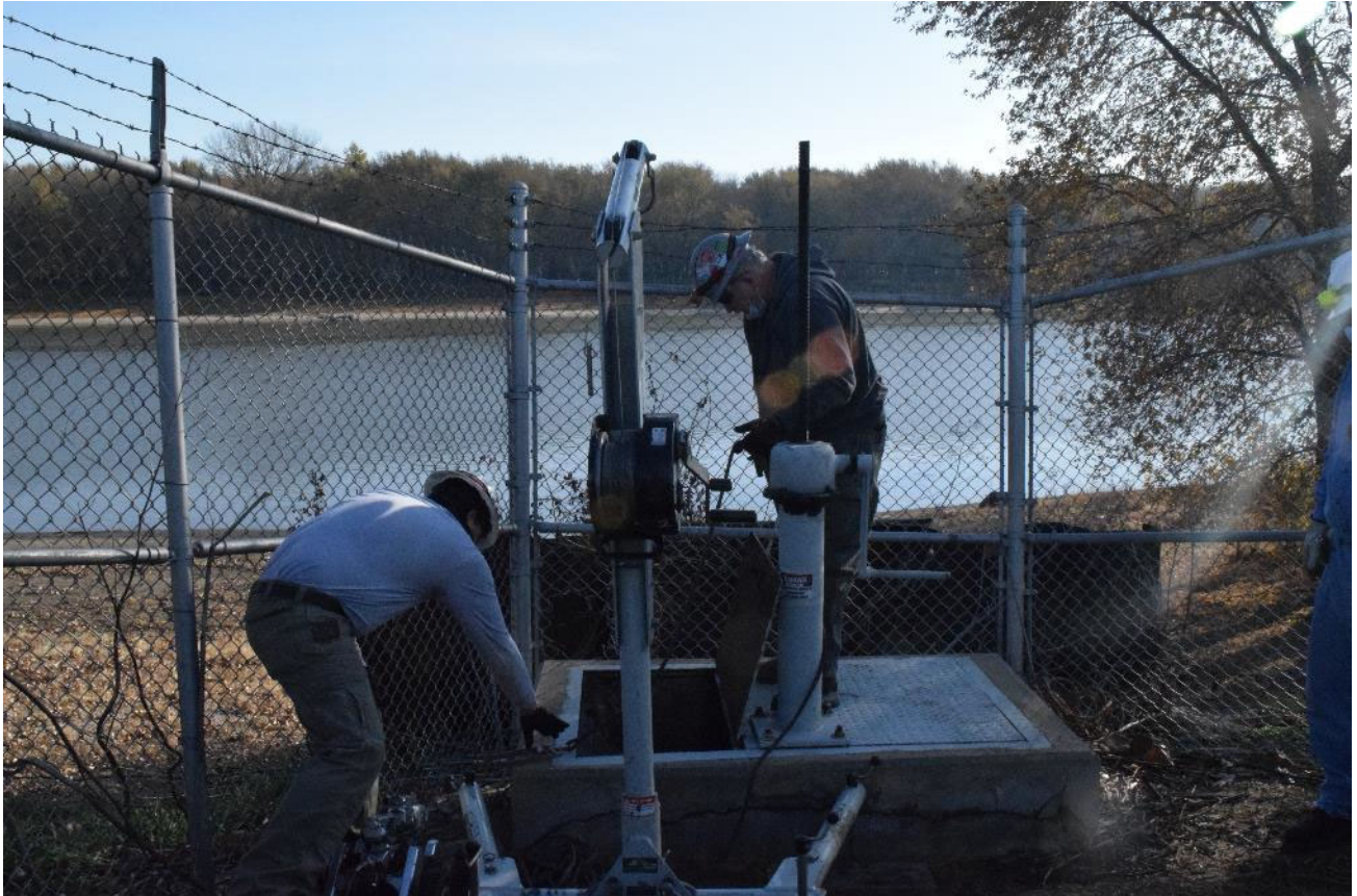
Outlet gate structure at Illinois River
