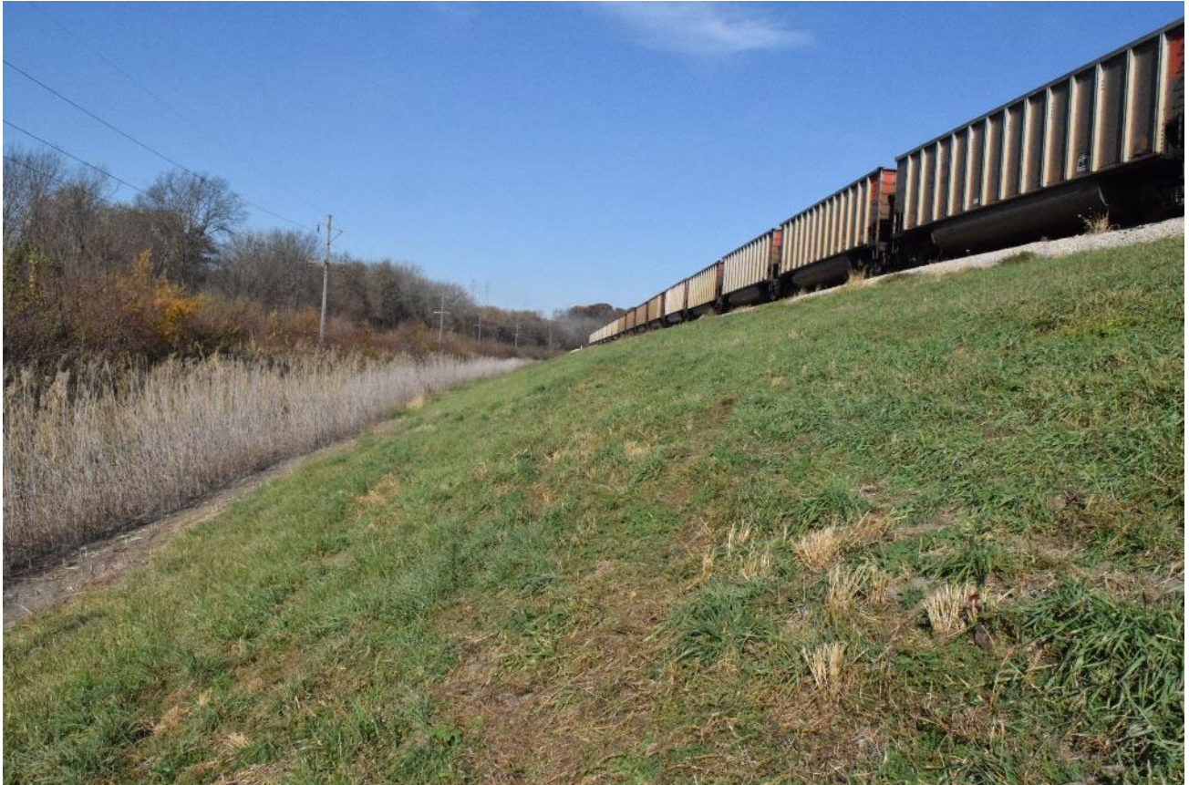
West side downstream slope
