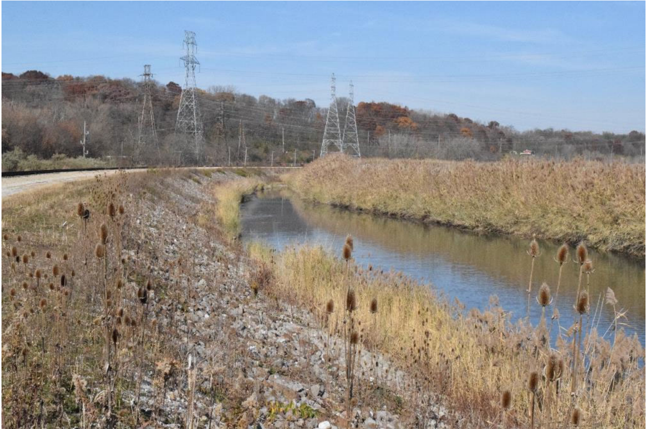
West side upstream slope
