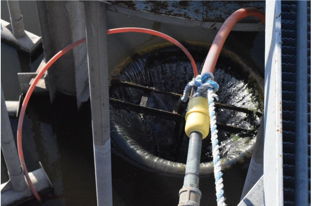
Pond outlet structure
