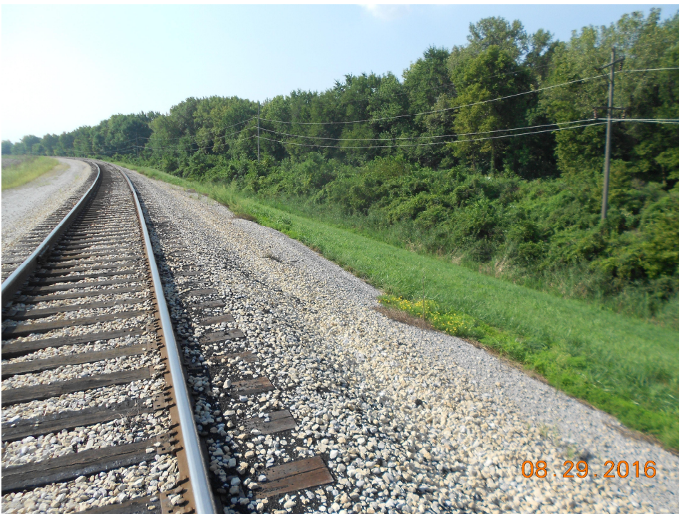
Figure E.4: Photo of Surficial Movement Area after Repairs
