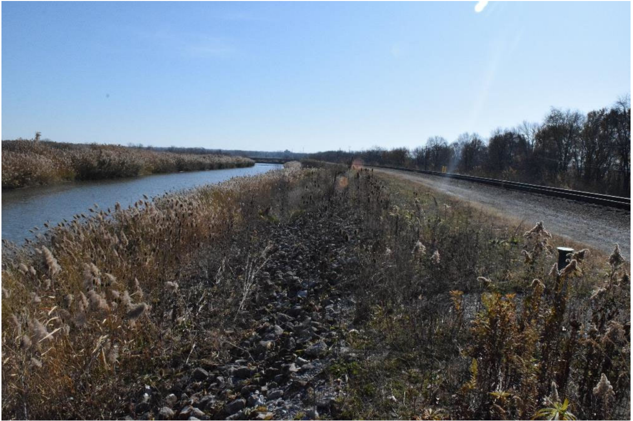
West side upstream slope
