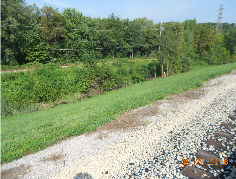
Figure E.3: Photo of Surficial Movement Area after Repairs
